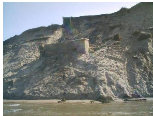
Figure 8 The Pillbox in 2004 following the dune collapse
