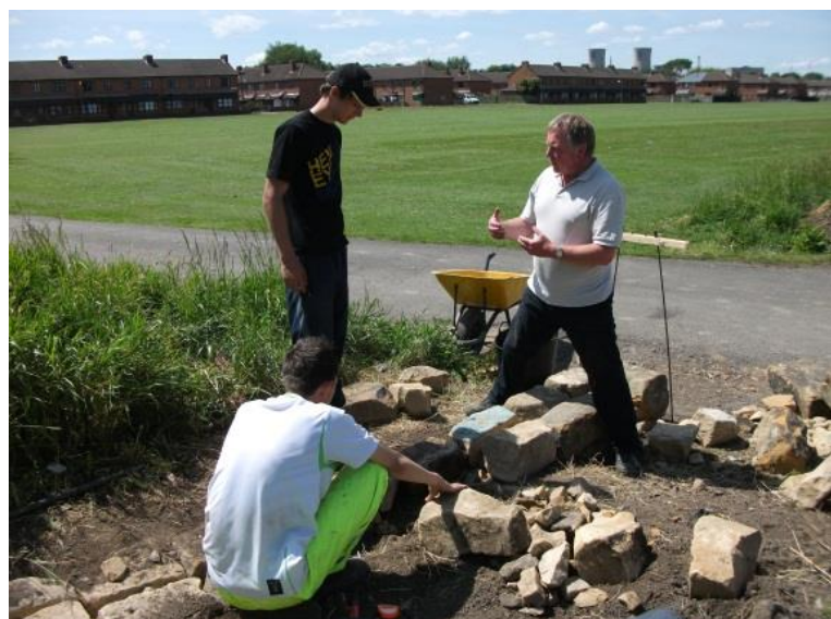
Figure 28 Dry Stone Walling © Know How North East
