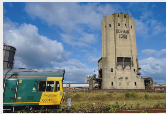
▲ Dorman Long Coal Tower
